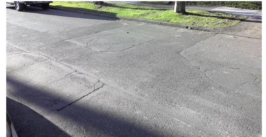
Restored trench opening on N Fowler, North of Lombard
