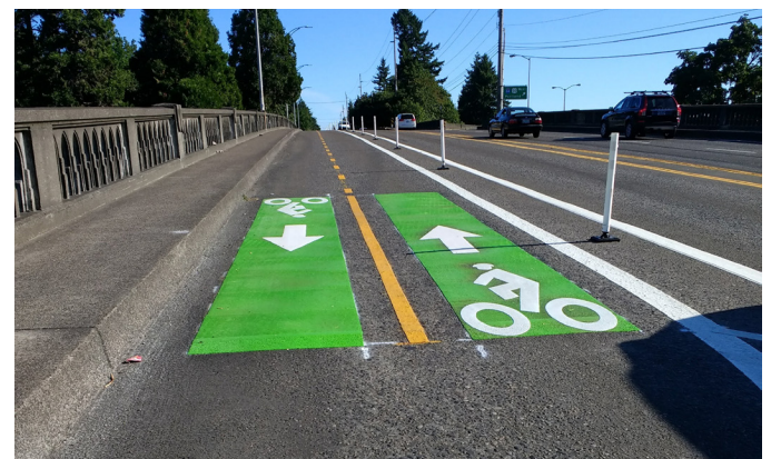
Two-way bike lane design near the sidewalk ramp
