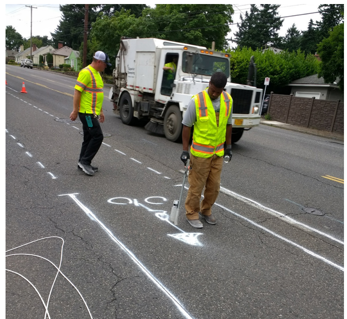
PBOT crews painting layout lines on NE 102nd Ave.
