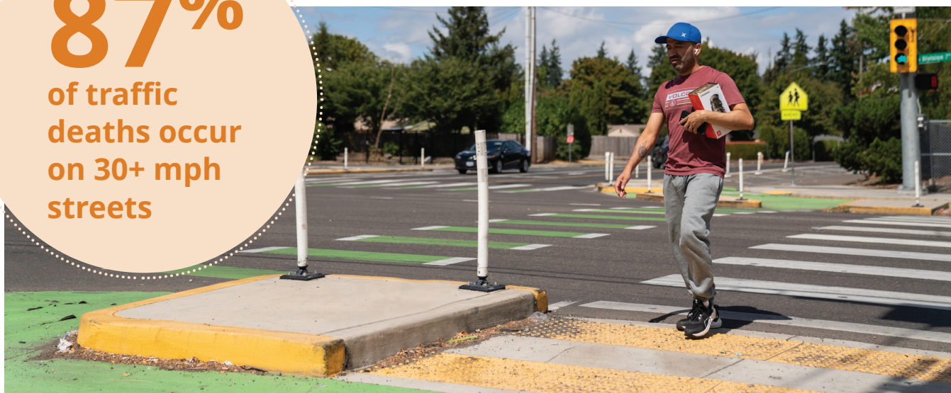
Figure 8. A new protected intersection in Southeast Portland designed to shorten the crossing distance and improve safety for people walking, biking, and rolling.
