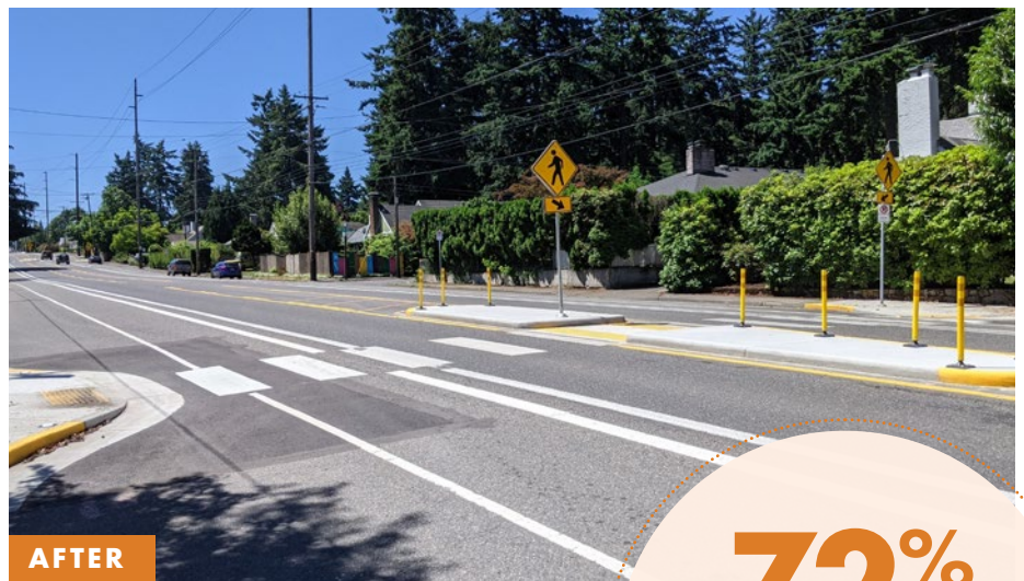
AFTER NE 102nd Avenue at Shaver Street, looking south, after the lane reconfiguration project in 2019. The street space is allocated to parking on both sides with curb extensions at the crossings, a buffered bike lane in each direction, one travel lane in each direction, and a center turn lane with median islands at pedestrian crossings.
