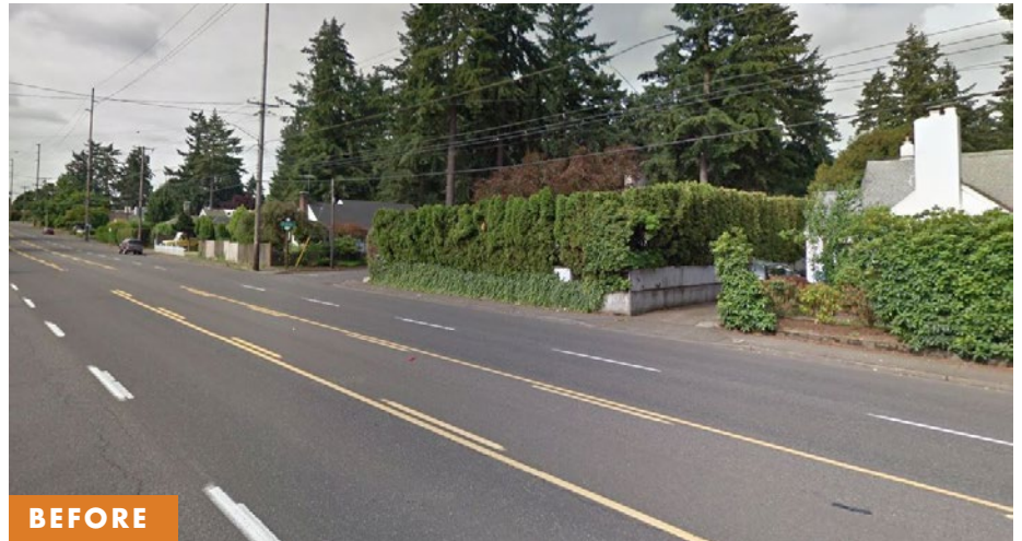
BEFORE NE 102nd Avenue at Shaver Street, looking south, before the lane reconfiguration project in 2019. The street space was allocated to parking on both sides, two travel lanes in each direction, and an open center-turn lane.
