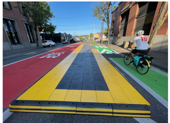
Transit platform at SE Hawthorne Boulevard and 6th Avenue
