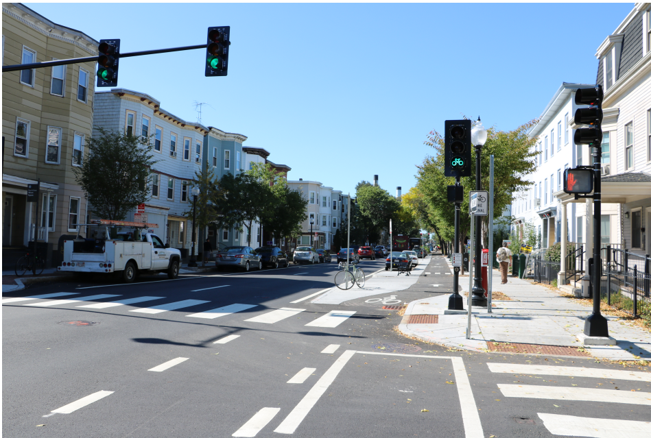
Sidewalk level separated bikeway Western Ave, Cambridge MA
