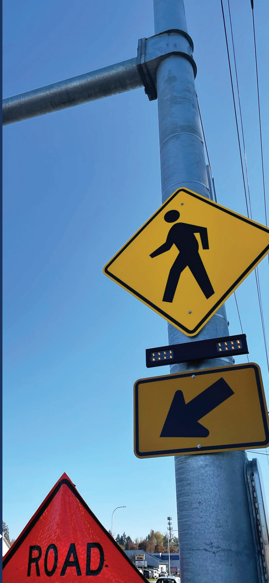
New RRFBs were added at Boardman and Hull.
