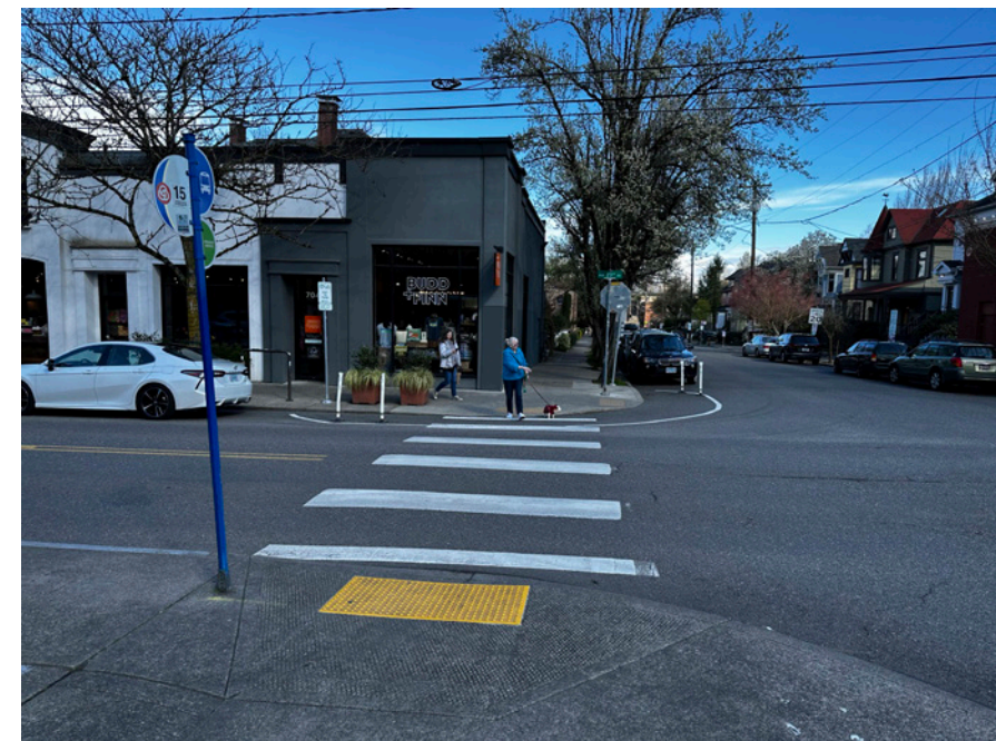
PAINT AND POST CURB EXTENSION WITH PLANTERS
