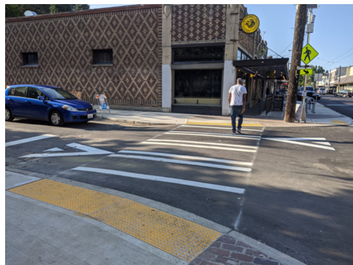
ALIGNED ACCESSIBLE CURB RAMP
