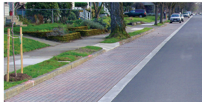
PERMEABLE UNIT PAVERS
