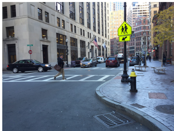
BUILT CURB EXTENSIONS
