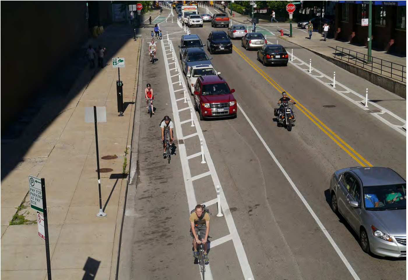
Figure 11. Parking protected bicycle lane on Kinzie Street in Chicago. Design used both parked cars and delineator posts for separation.
