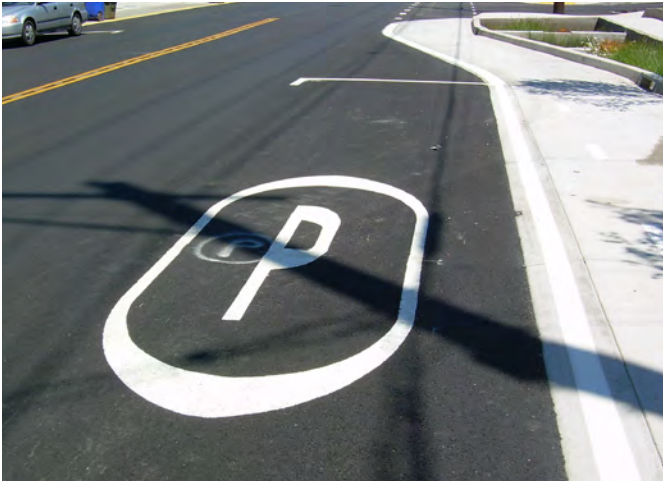
Figure 13. Parking stall on NE Cully Boulevard, Portland, OR.
