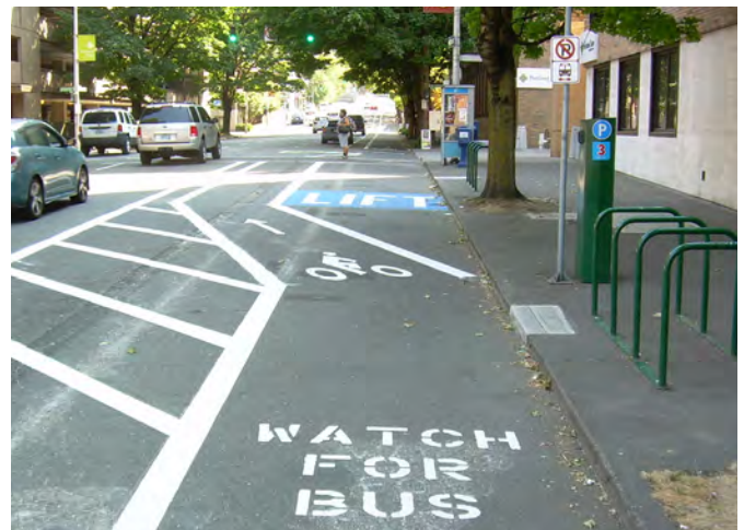
Figure 16. Curb access with a painted parking-protected bicycle lane (SW Broadway, Portland). Elsewhere, the areas shown hatched is for car parking. To allow LIFT vehicles to the curb the bicycle lane deflects around the LIFT access area (marked in blue). When a vehicle is servicing the stop a buffered bicycle lane remains. When no vehicle is there people bicycling can maintain a straight course. This was implemented where dimensions were: 8 foot – 3 foot – 7 foot (parking, buffer, bicycle zone respectively).
