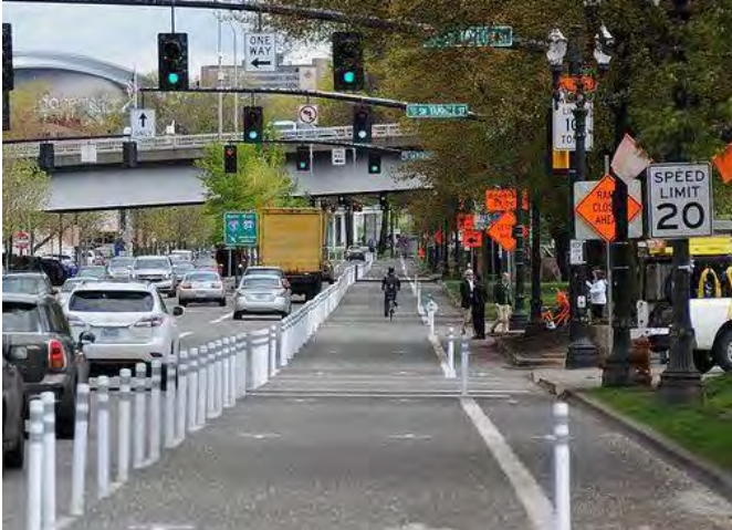
Figure 7. “Better Naito” showing spacing of 12 feet between delineator posts. The posts are mounted directly on the lane line, adjacent to an 11’ travel lane; an effective 10’ travel lane with a 1’ shy distance. (Photo: bikeportland.org/J. Maus)
