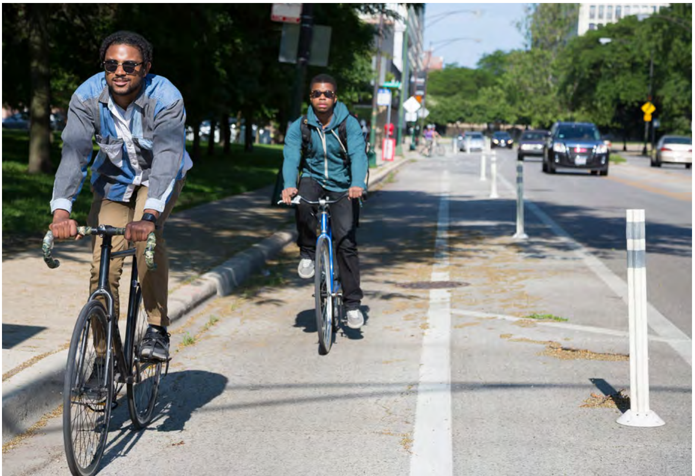
Figure 5. Bikeway protected with plastic delineators in Chicago.
