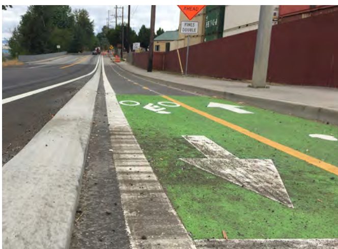
Figure 9. Traffic separator protected lane on N Burgard Rd, Portland. Source: Matt Ferris-Smith, PBOT
