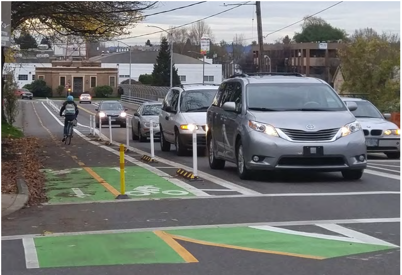
Figure 6. Parking stops and delineator post barrier on two-way bikeway on NE 21st Avenue in Portland.
