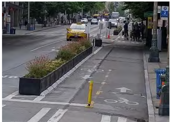
Figure 10. Linear array of planters on Seattle's 2nd Avenue (two-way) bikeway
