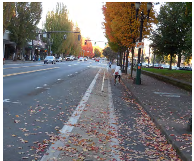
Figure 14. Colored buffer zone with delineators on NE Multnomah, Portland, OR. Current guidance would place delineators closer to the parking zone.
