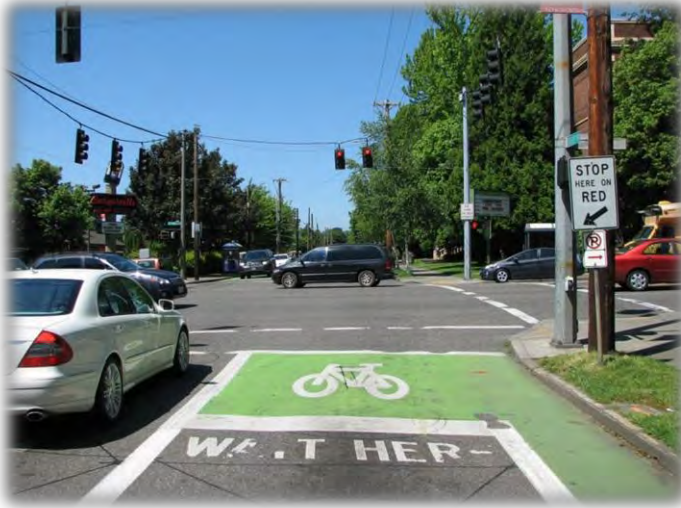
Exhibit 23 Example of a Bike Box at Powell Boulevard/26 th Avenue
