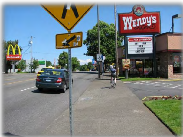
Exhibit 21 Example of Potential Bicycle/Pedestrian/Vehicle Conflict at Commercial Driveway
