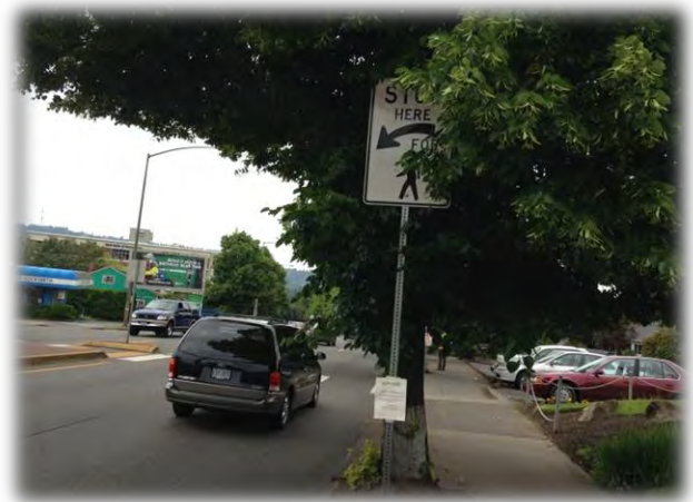
Exhibit 5 Signs Blocked by Trees
