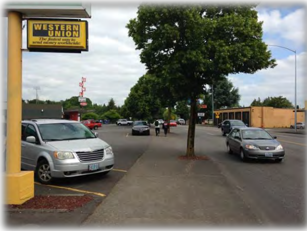
Exhibit 8 Limited Sight Distance Due to Trees on Horizontal Curve
