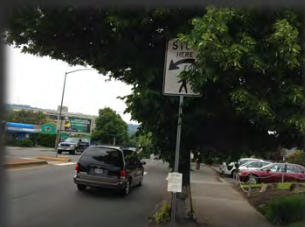
Signs Blocked by Trees
