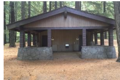
PCT trail improvements should include facilities at Toll House Park on the Oregon Bridge Head
