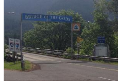
The Washington Bridge Head provides no clear pedestrian access to the bridge.
