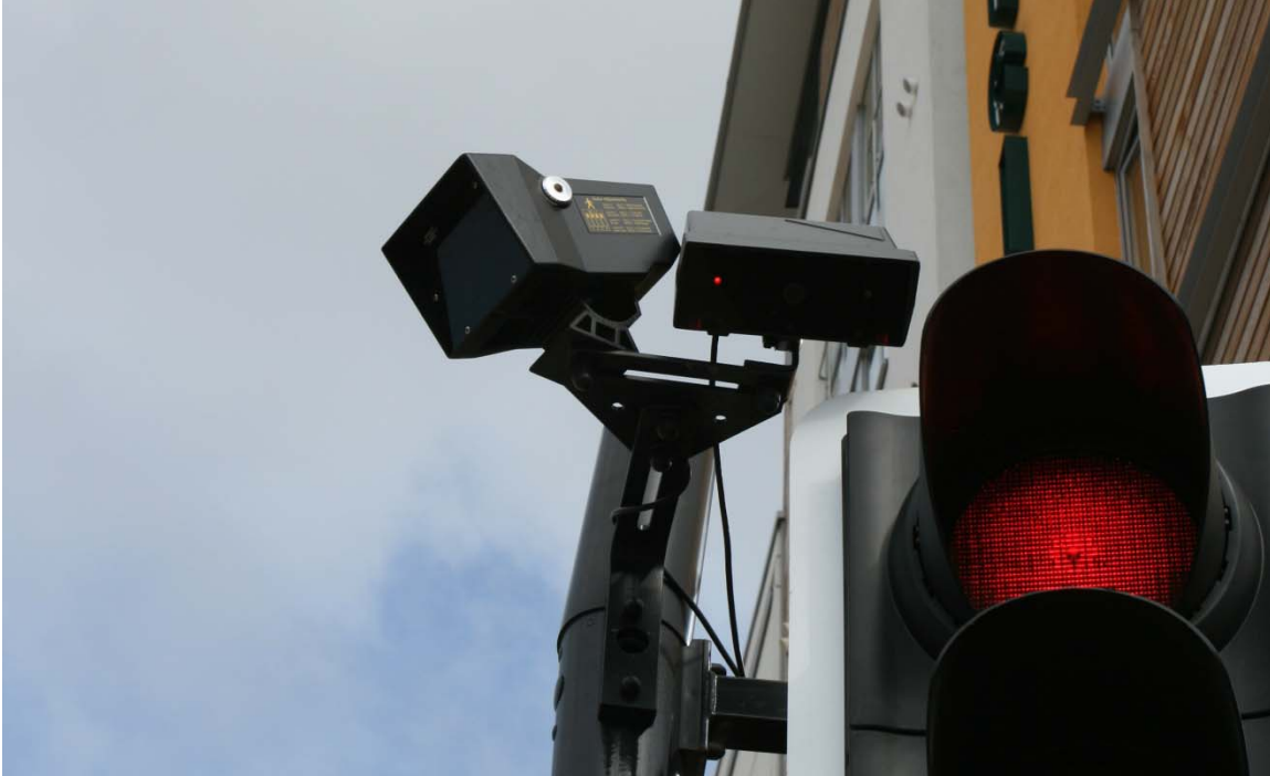
Figure 2. Automated Pedestrian Sensors are Used to Adapt Signal Timing for Pedestrians (Bristol, United Kingdom)
