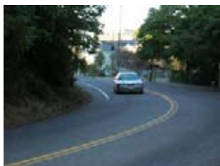
Substandard bike lane south of Sheridan
