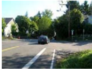
Poor sight distance as bike lane ends at Texas
