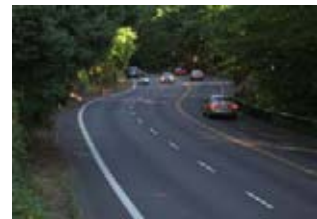
No downhill bike lane and narrow uphill bike lane between Barbur-Terwilliger
