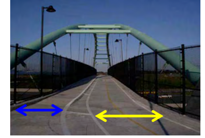
I-80 Ped/Bike Bridge Berkeley, CA
