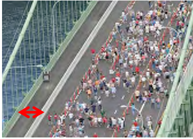
Tacoma Narrows Bridge Tacoma, WA
