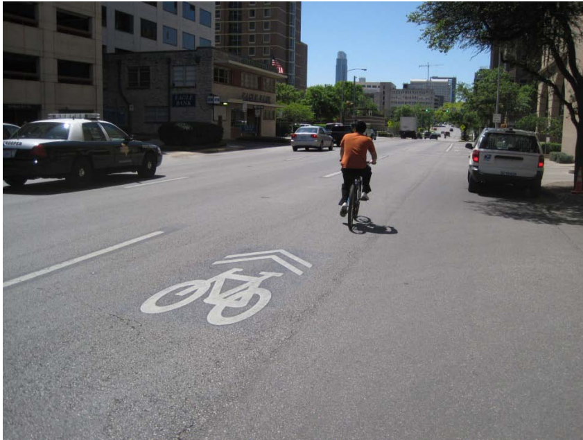
Figure 21. Central placement of sharrow resulted in thriving thermoplastic five months after installation.
