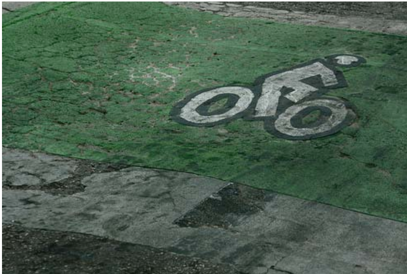
Figure 19. Poor quality of road led to the deterioration of the thermoplastic bike boxes on Speedway
